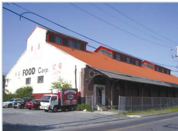
Former Philadelphia, Wilmington & Baltimore Railroad freight depot at Broad and Washington streets.
