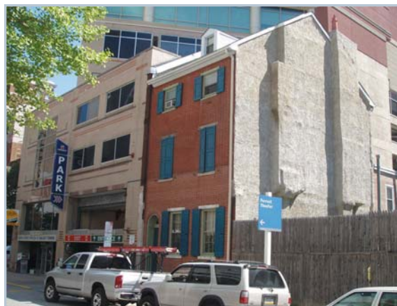
215 S. 9th Street. This property is the only remaining building in the William Strickland Home Row, a seven-building National Register listed historic district.
